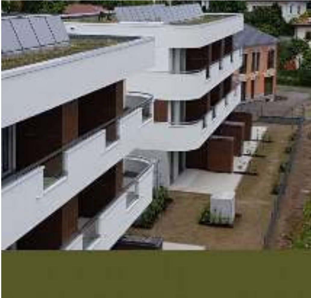
48 Apartment Houses built in Obert. (Germany) Building volume around 27.85m €
