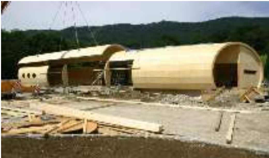
Restaurant built in Konstanz (Germany) Building volume around 730k €
