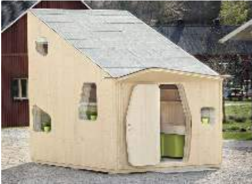
20 Student Houses built in Karlsruhe (Germany) Building volume around 450k €
